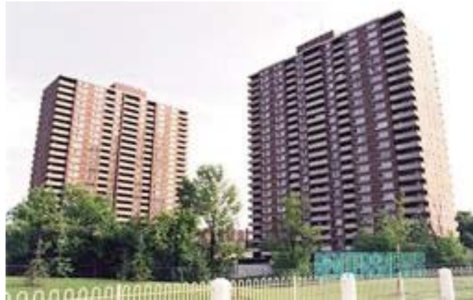
◀ The buildings at 2667 and 2677 Kipling Avenue in Etobicoke are one site of the Mayor’s Tower Renewal. Source: rentersnews.ca
